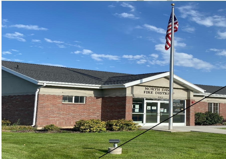
West Point Station 41 NDFD Headquarters
